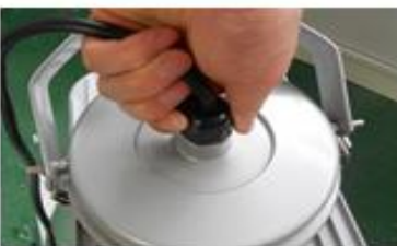
8. Fix the waterproof connector and connect to AC cable
